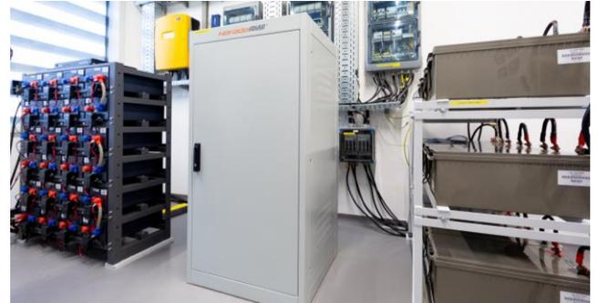
Figure 2. HyStore indoor batteries: Advanced Lead Carbon, Lithium Iron Phosphate and GEL Lead Acid
